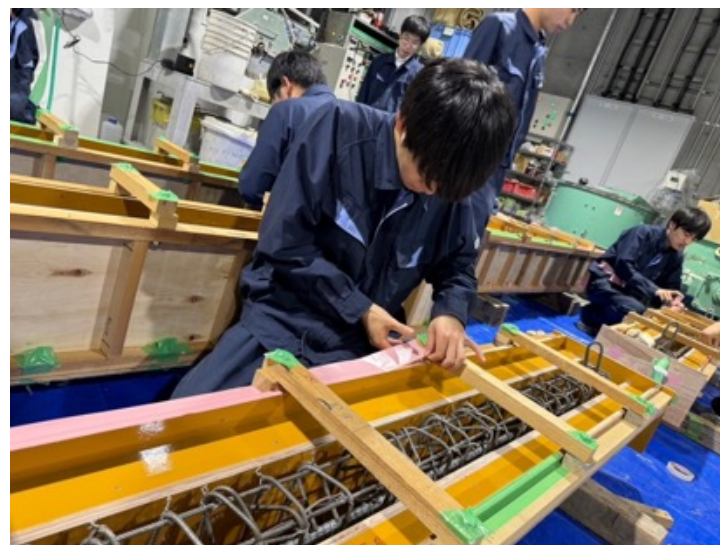
打設前 Before casting
