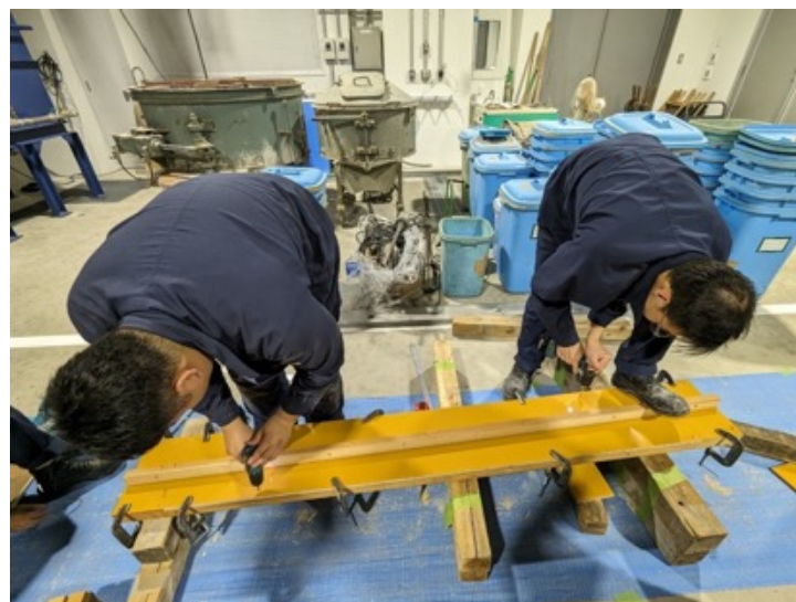
型枠作成 Making formworks
